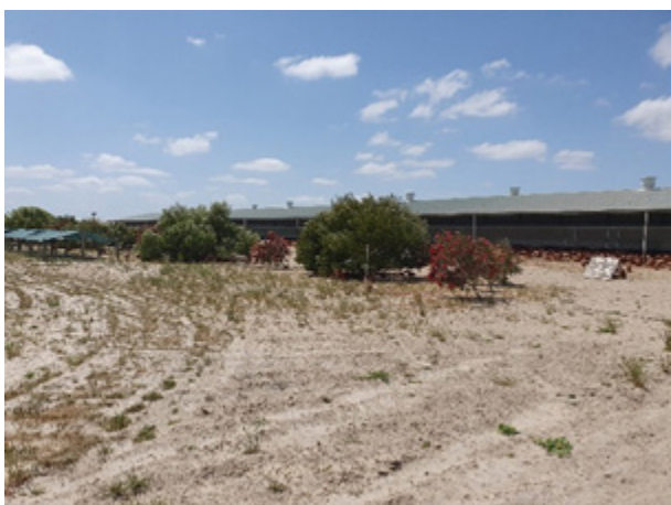
A combination of fixed canvas shelters, portable, home-made shelters, and trees are used on range areas.
