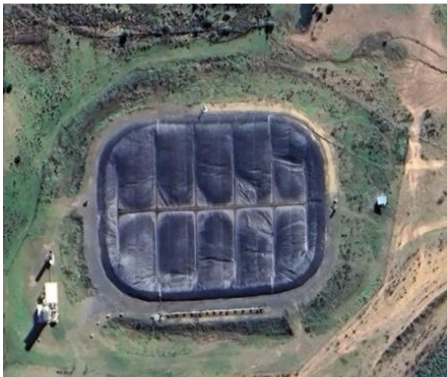
Figure 13 Covered anaerobic pond with renewable energy generation constructed under a third party build-own-operate model
