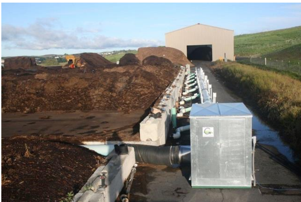
Figure 5 Forced aeration of a static pile
