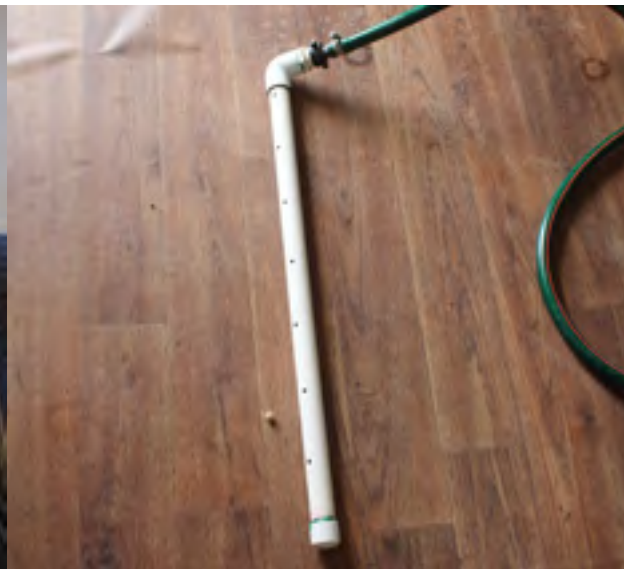
Photograph 13: Centralised Gas Delivery System
