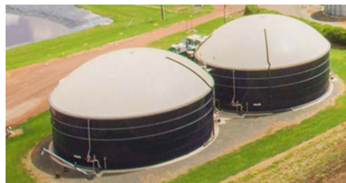
Figure 12: Example of an engineered above-ground digester Source: BettaPork
