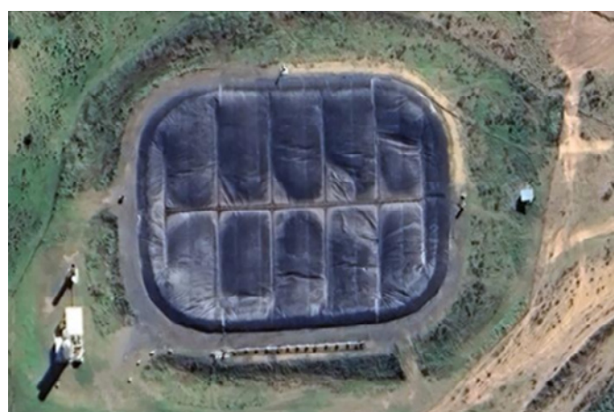
Figure 13: Covered anaerobic pond with renewable energy generation constructed under a third party build-own-operate model Source: Google Earth.
